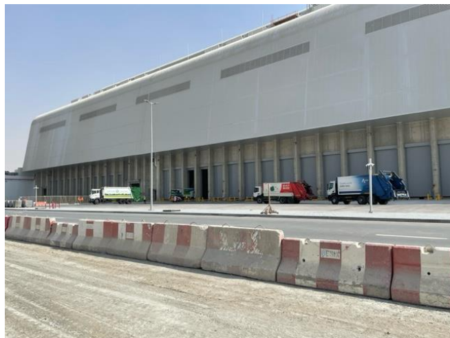
Waste delivery vehicles maneuvering into position in block 2.
