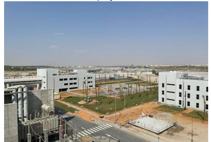
The administration and accommodation buildings have been approved for use by the authorities in August
